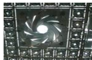
Fig .3. The dynamic circular shutter adopted from the traditional mashrabiya
