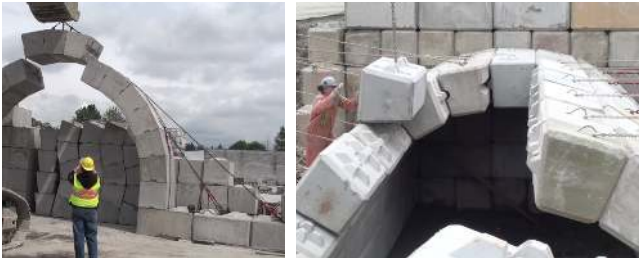
Figure 2: The Arch-Lock system [Drew 2013] is used to construct a simple arch (left), and a barrel vault (right). [Copyright photographs: Lock-Block Ltd. 2013]
